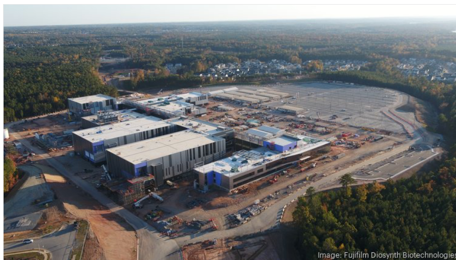
Aerial view of the Fujifilm Diosynth Biotechnologies facility in Holly Springs.
